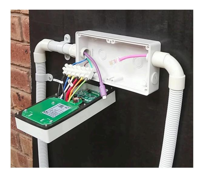
11. All power supplies to the CET-HD-PM2 must be protected by an upstream protection device (or a combination of devices) with a trip current of 32A or less and an earth-leakage trip current of 30mA or less.
