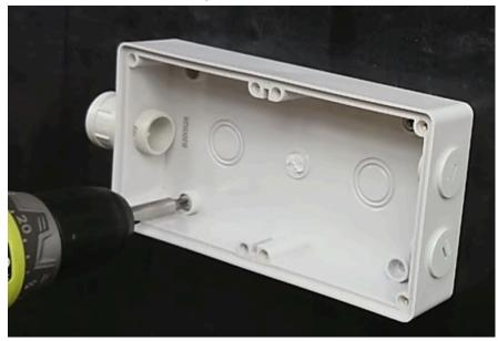
4. Ensure that the enclosure base is mounted flat against the surface and that the base is not warped. If the enclosure base is warped the lid will not seal to the base correctly and the product IP rating may be compromised:
