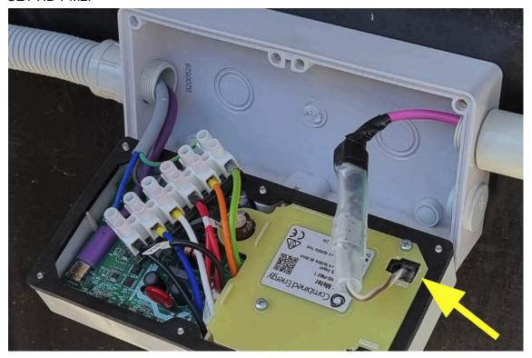
Terminate the **brown wire** from the Inverter to the data positive "+" INV terminal of the RS485 filter, and the brown-white wire to the data negative "-" INV terminal.
