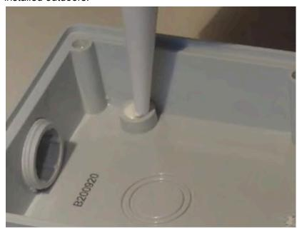
7. Press the included plastic screw covers into the mounting screw holes:
