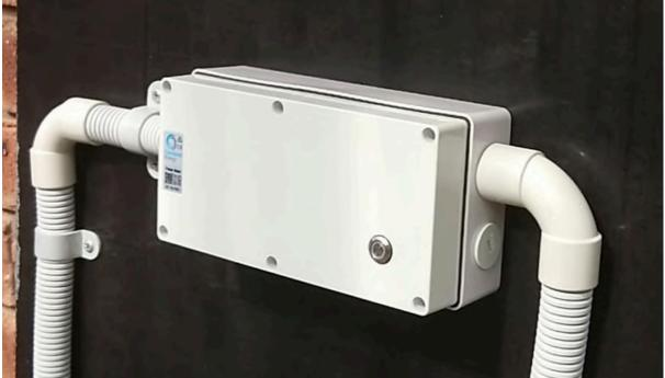
16. Once the lid has been secured, apply power to the CET-HD-PM2 and check it is operating correctly. The button will illuminate when power is applied and turn red (if there is no EMU in range) or green (if the site EMU is installed and communicating with the CET-HD-PM2 correctly):
